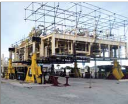
Assembling an Offshore Platform Oil Rig Module
