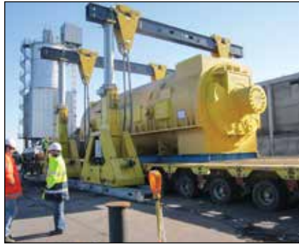
Turbine Lift and Load-in at Shipping Port
